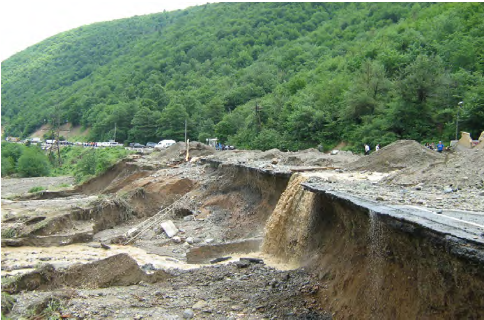
Photo 4.4.1. On 18 June 2011 more than 100 mm of rainfall happened during 2 hours in Chumateleti. As a result 6 persons died and more than 100 households were flooded and destroyed by the mudflow. Mud torrent was not recorded on this territory before.
