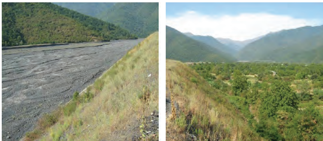
Photo. 4.3.4. Dam arranged to protect the bank of the Duruji
