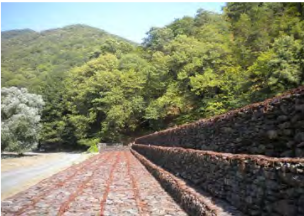
Photo. 4.3.3. River dike protection on R. Duruji coast
