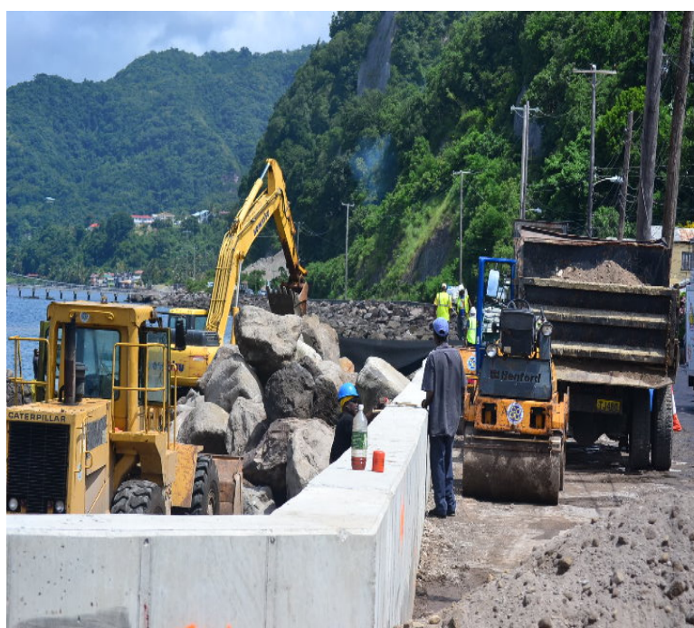
Photo 5.5 Pointe Mitchel Sea Wall under construction
