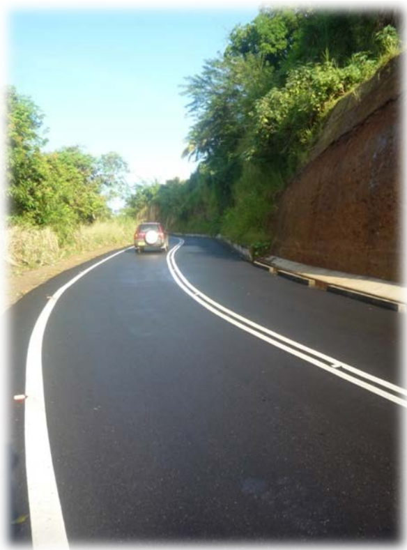
Photo 5.1 Recently rehabilitated Bath Estate- St Aroma link road
