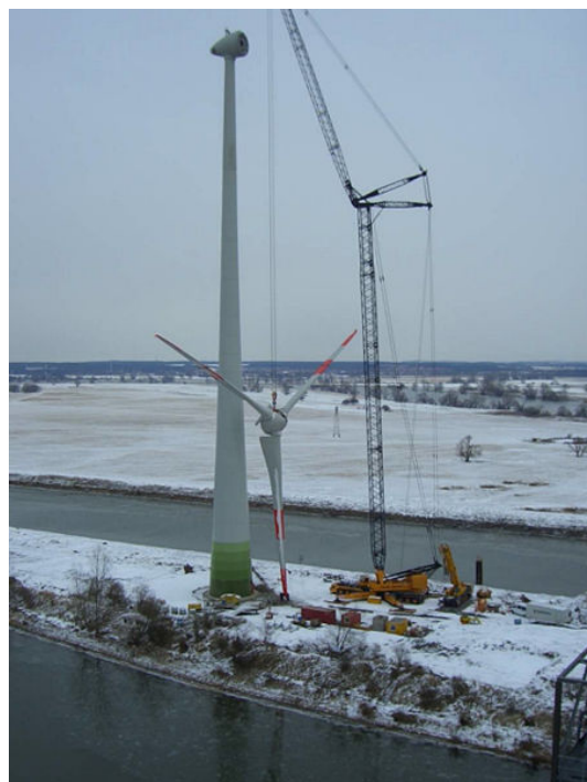
Figure 3.7: Erection of an Enercon E70-4 in Germany (Wikipedia)
